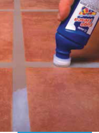
Floor in terracotta treated with Fuga Fresca
